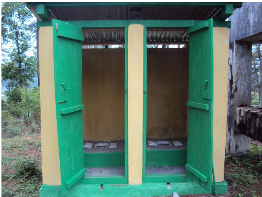
TOILET FACILITY FOR OPD
